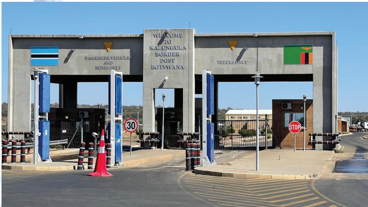
Exit Gate at Botswana Kazungula Bridge OSBP
