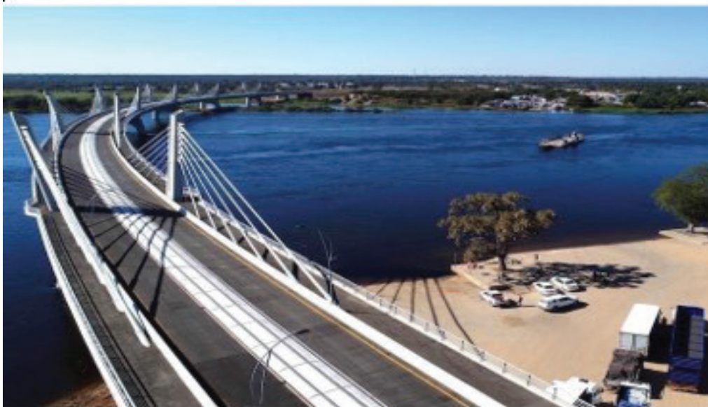
Ultra-modern Kazungula Bridge connecting two countries (Botswana and Zambia)
