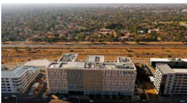
BURS aerial view
